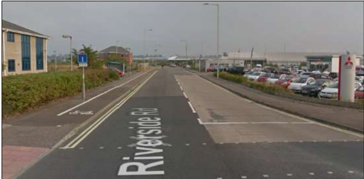
Figure 3.17: Riverside Road Segregated Footway / Cycleway (Source: Google Maps Streetview)
