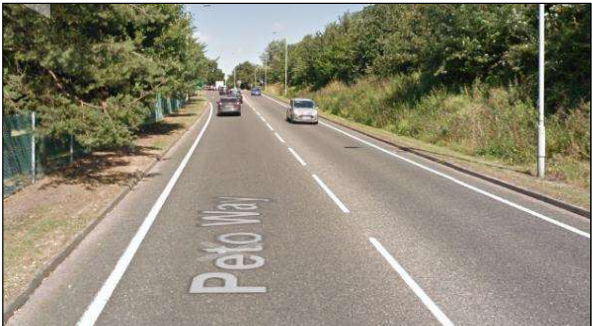
Figure 3.7: Peto Way Informal Footways (Source: Google Maps Streetview)
