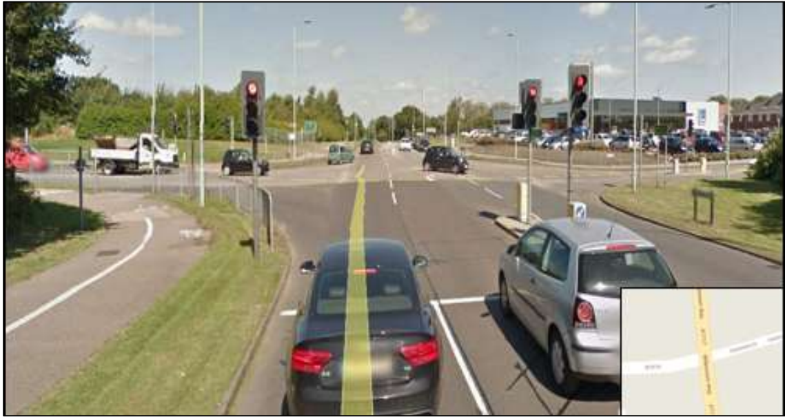
Figure 8.26: A1117 Millennium Way / B1074 Somerleyton Road signalised junction (Source: Google Maps Streetview)
