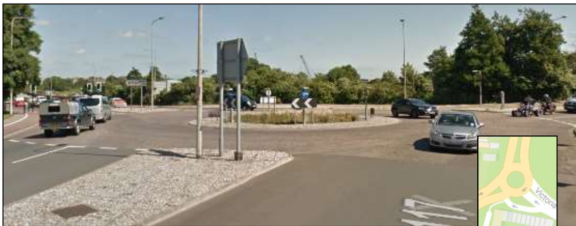
Figure 8.16: A1117 Saltwater Way / A1117 Bridge Road / B1531 Victoria Road roundabout (Source: Google Maps Streetview)
