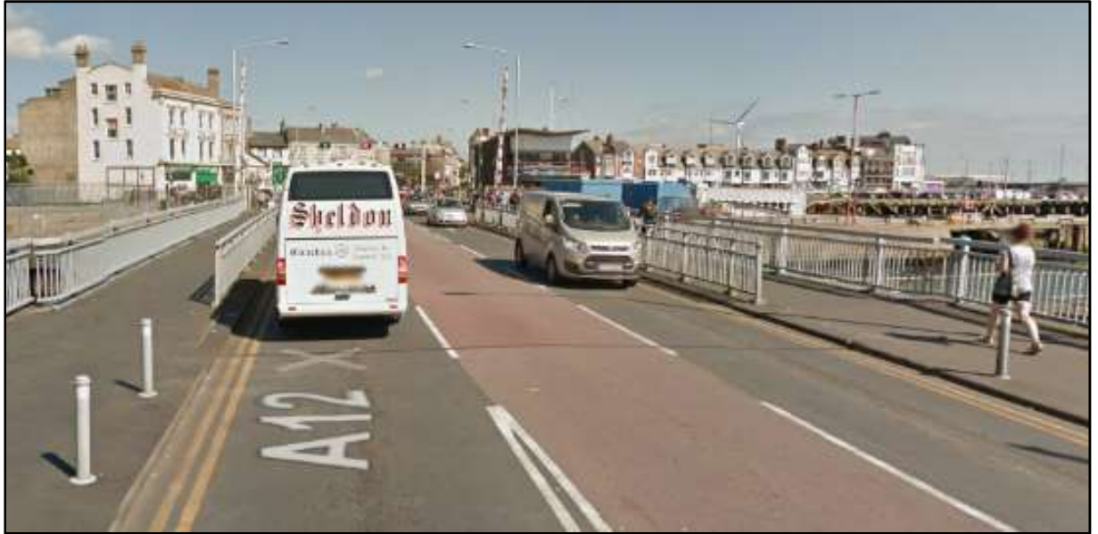
Figure 3.8: The A47 Bascule Bridge footpaths (Source: Google Maps Streetview)
