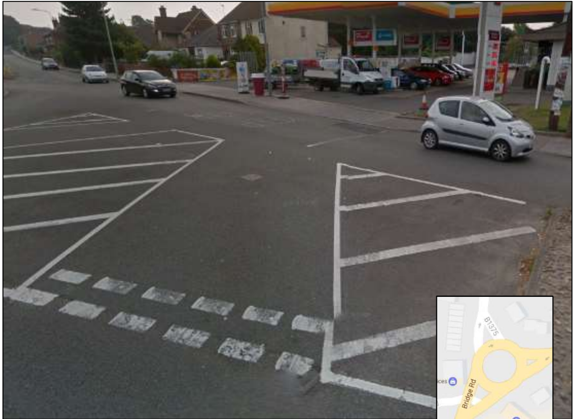
Figure 8.17: Priority junction for vehicles exiting the petrol station onto the northbound approach of the A1117 Bridge Road (Source: Google Maps Streetview)
