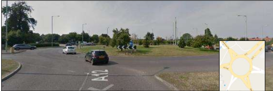
Figure 8.14: A12 Tom Crisp Way / A12 Bloodmoor Road / A1145 Castleton Avenue roundabout (Source: Google Maps Streetview)
