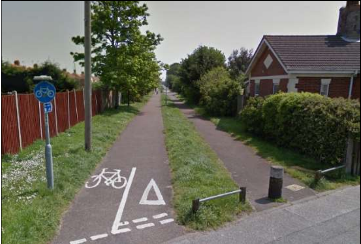
Figure 3.16: Kirkley Run Segregated Footway / Cycleway (Source: Google Maps Streetview)
