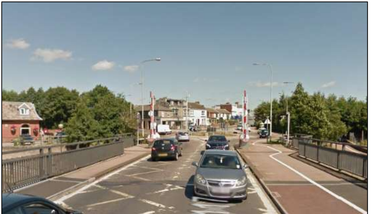
Figure 3.9: Mutford Bridge Segregated Footway / Cycleway (Source: Google Maps Streetview)
