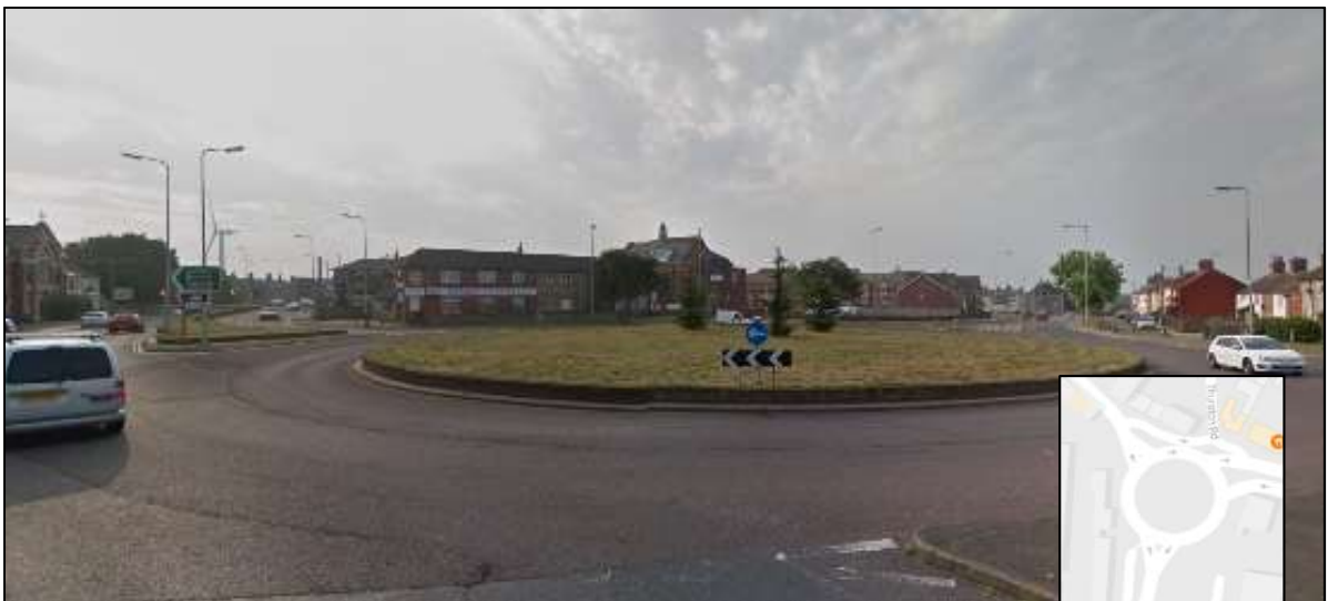
Figure 8.2: A12 Katwijk Way / A1144 St Peter's Street roundabout (Source: Google Maps Streetview)
