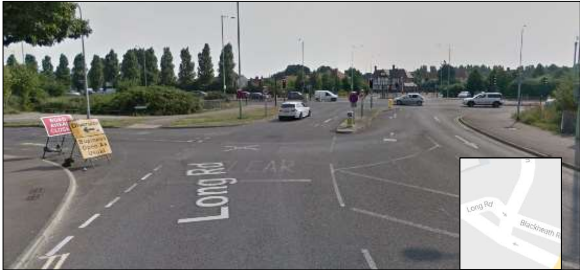
Figure 8.12: Kirkley Run / Blackheath Road / Long Road priority junction (Source: Google Maps Streetview)
